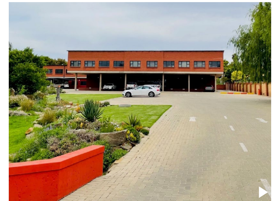
Warwick Wealth Bloemfontein Offices
